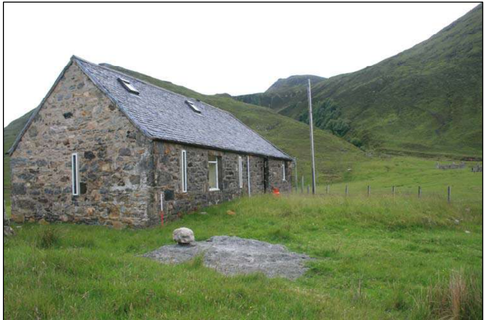
Fig 15. Threshing barn, 449, now a holiday cottage, and horse gang 448 at Corrieveuc from the NW
